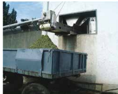
Vegetable processing wastewater screening prior to being treated in a multi-stage Submerged Aerated Filter Plant.
