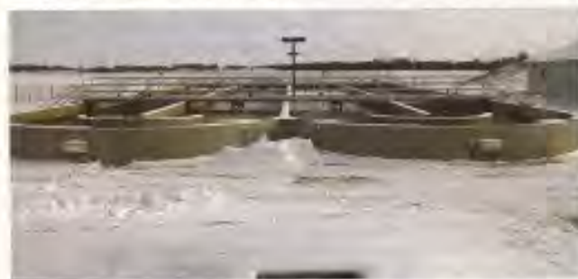
A view from the west end of the two-ring oxidation ditch at Dawson, MN. The DO probes are mounted in the foreground in the corner of each ditch near the center dividing wall.
