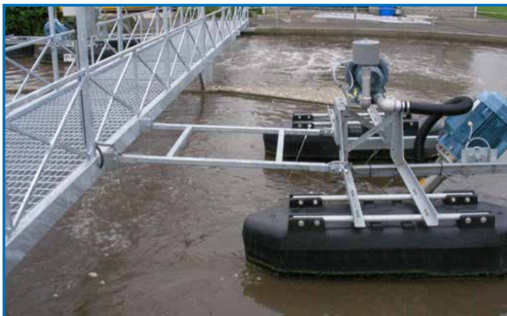
3.7kW Tritons® fixed on a tri-pontoon float. The Triton® can be bridge or side-wall mounted.
