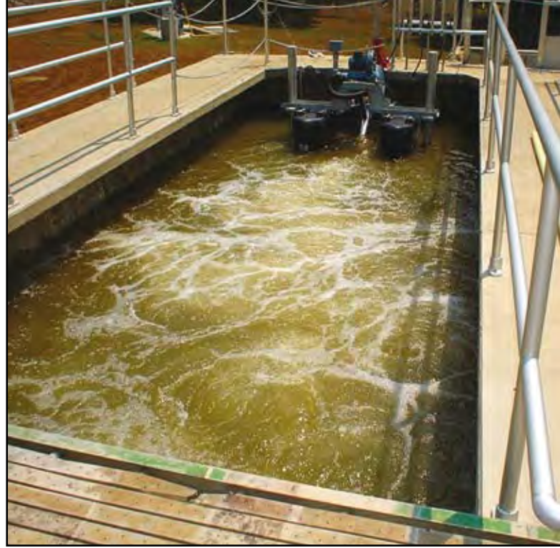
The Triton dual-function aerator/mixer provides process flexibility to nitrify and de-nitrify as well as facilitate biological phosphorus removal by changing controls to allow for anoxic mixing steps during the cycles.
