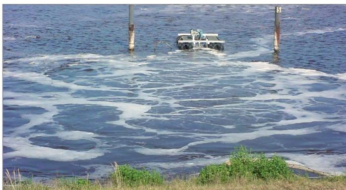
Factors that affect aeration oxygen transfer and wastewater treatment performance efficiency include bubble size, hang time and complete mixing of a basin to prevent dead spots and short circuiting. The process aerator/mixer's ability
