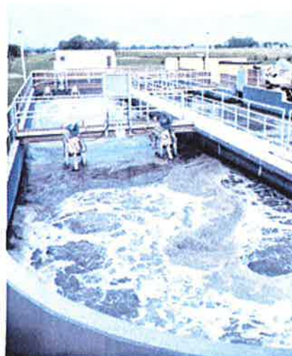
A ditch close-up shows bridge-mounted units.
