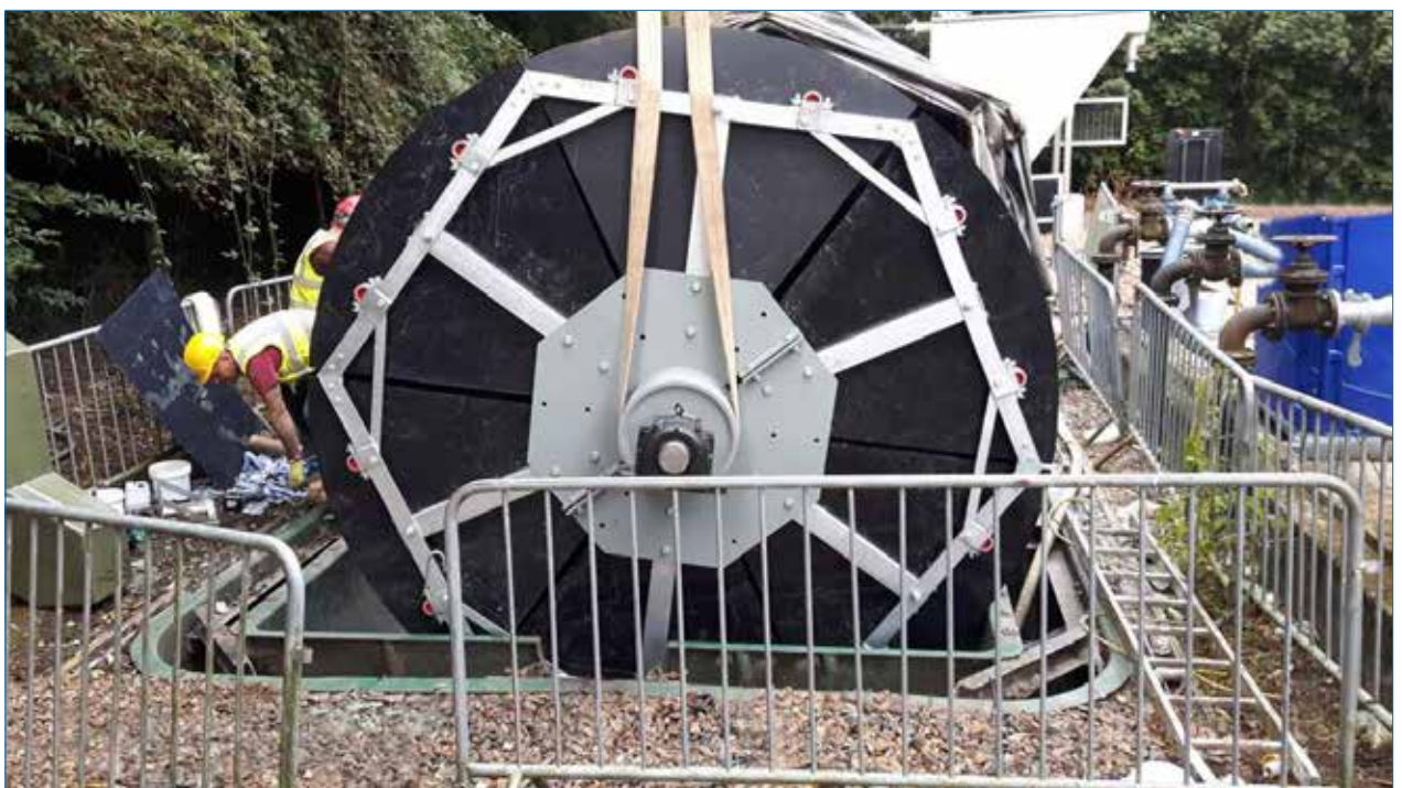
Anglian Water, Brinkley
