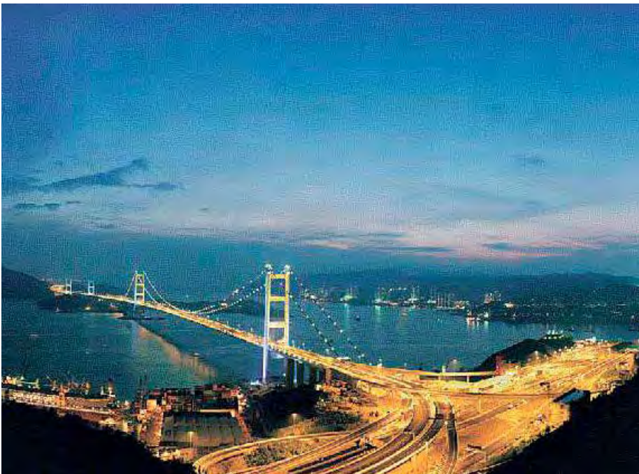
KEE Process install RBC plant for new residential development facing the Tsing Ma Bridge, Hong Kong.
