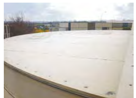
Top roof section of cover
