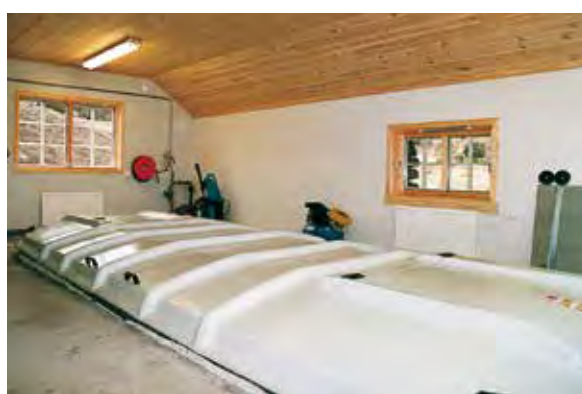
BioDisc package single piece plant including phosphorus removal to under 1mg/l.
