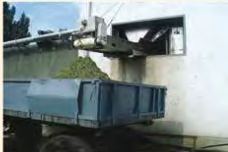
Effluent screenings from vegetable processing plant
