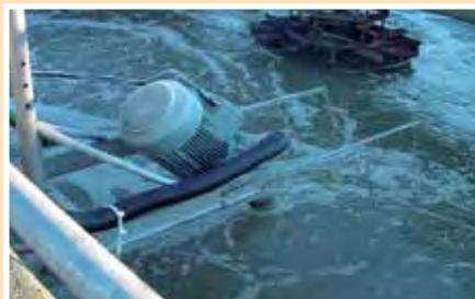
Plant upgraded with no downtime in less than a week with four KEE Tritons® bolted to the side and one is seen here in operation.
