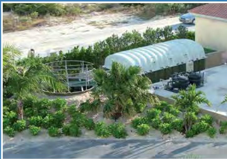
*KEE Managed Flow RBC Module Model DC17 and a modular fibreglass hopper bottom final settlement tank installed at the Five Star Grace Bay Club.*
