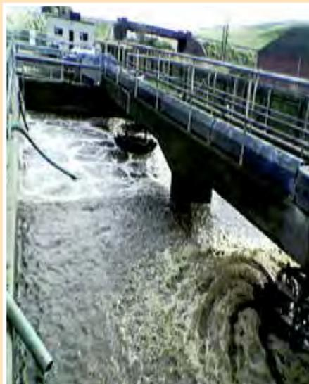
Existing Aeration system in need of upgrading as only one surface Aerator was operating.
